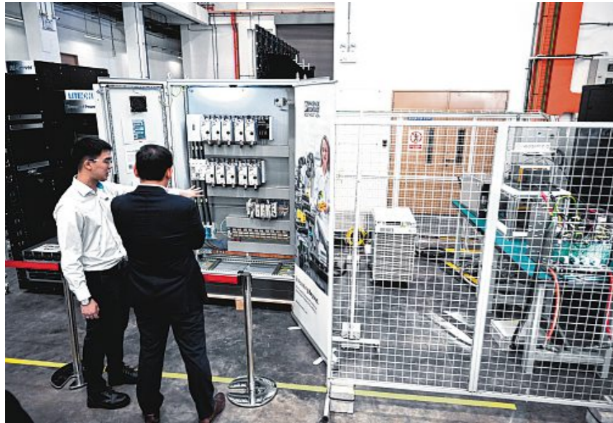
The new HVDC infrastructure will allow data centres to support ultra-high-density racks exceeding 1 MW with higher reliability and lower costs. PHOTO: ST
